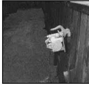
Septic Tank with US-900 & Wedge Bracket
