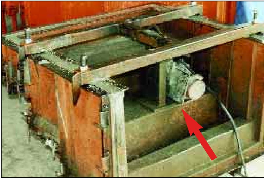
3-Step Form using US-900 Electric with UW-2 Wedge Bracket.
