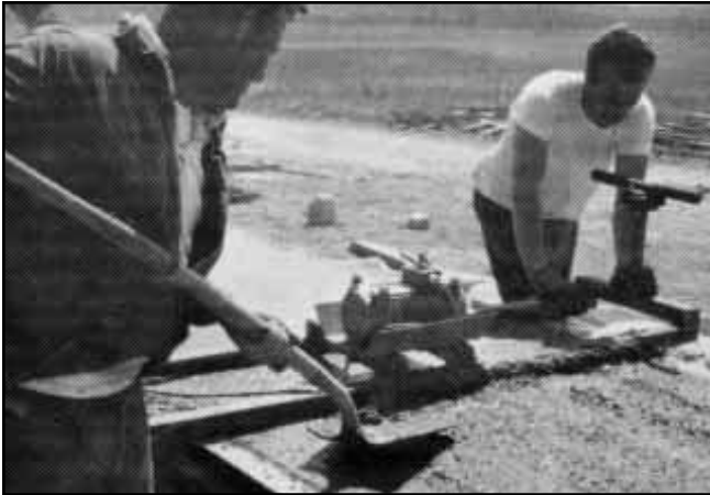
Screed made from 2" x 4" steel tubing and Model 2P-450 Electric Vibrator .
